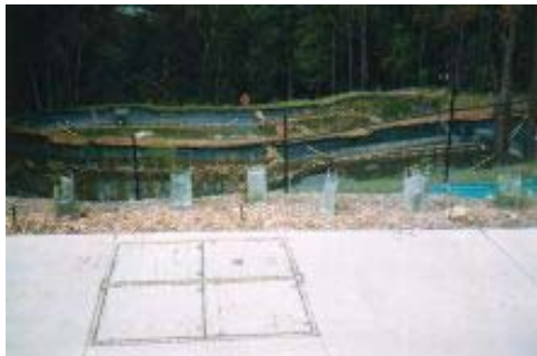
Above: A SurfSep screening motorway run-off with a series of man made detention ponds in the background.
