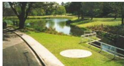
Above: A large SurfSep (200 ha +) protecting a series of natural retention wetlands.
