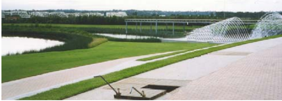
Below: A SurfSep installed upstream of a retention / detention pond. The water feature not only provides a visual public display but also increases the dissolved oxygen in the water and also provides good circulation of flow throughout the reed beds.
